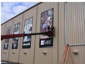
Installation of large banner stretch frames. Size: 23 ft x 11 ft
